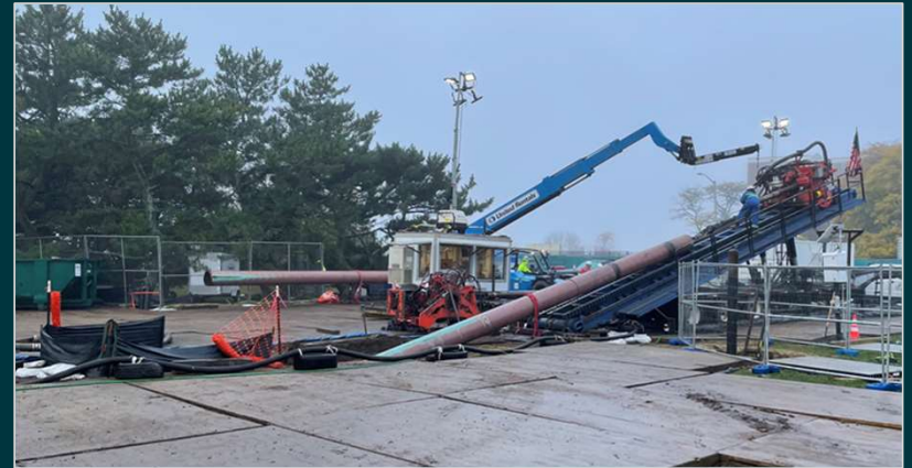
Installation of Casing Pipe
