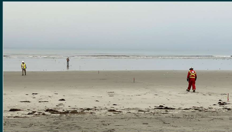
Beach Layout Of HDD Monitoring Grid
